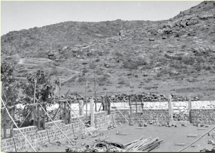
Old Dining Hall Construction
