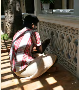
Repairs on the Nirvana Room Grillwork
